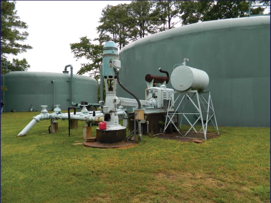
WATER WELL 1 AND RIGHT ANGLE DRIVE
