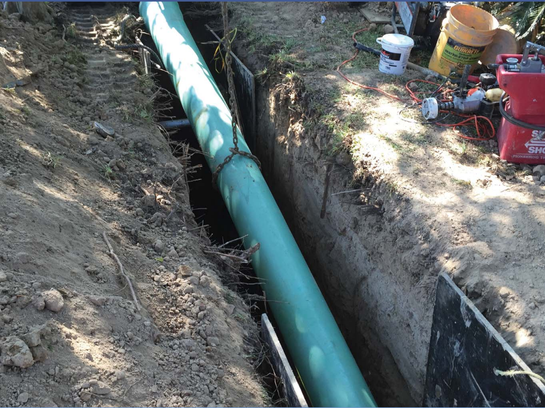
NEW SANITARY SEWER LINES AND SERVICES
