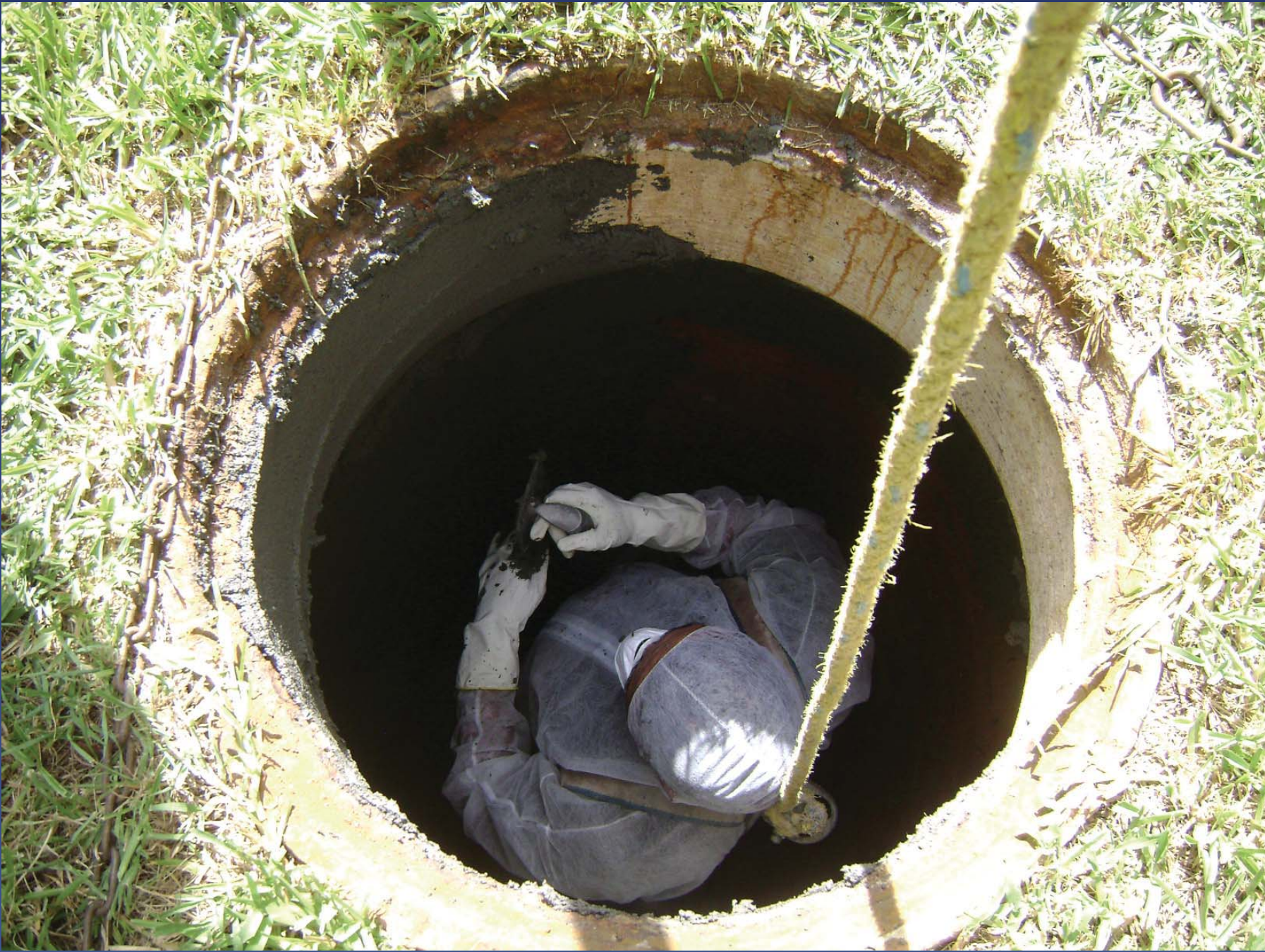
MANHOLE REHABILITATION
