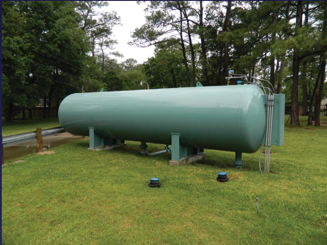
5,000 GALLON HYDRO-PNEUMATIC TANK
