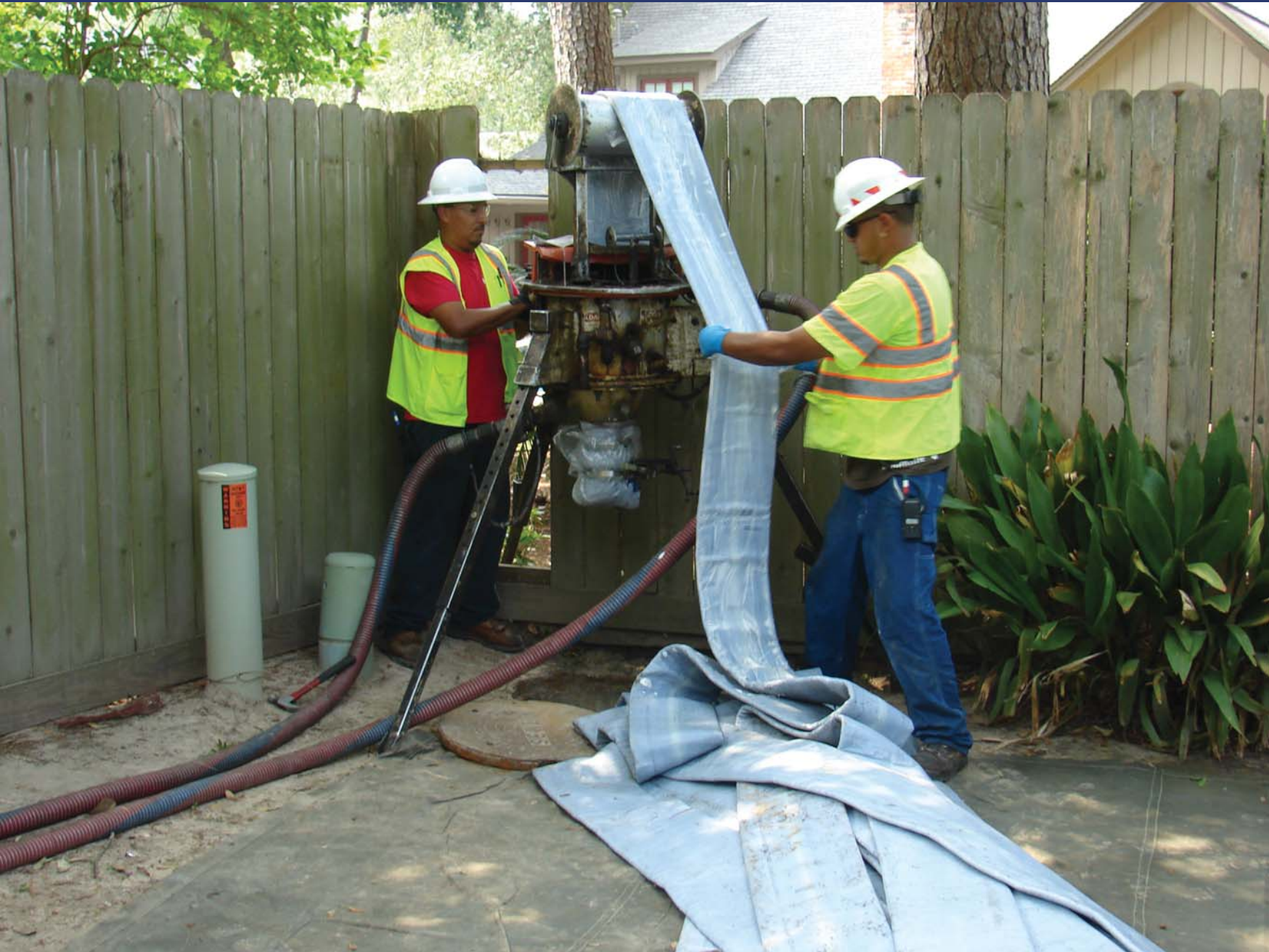
CURED-IN-PLACE LINING (CIPP)
